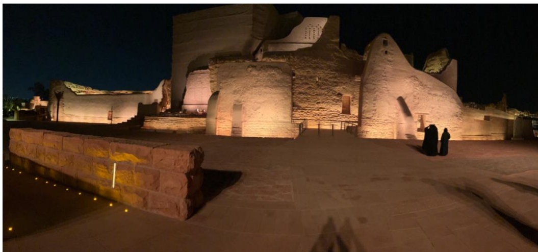
Compound Project centered on the Preservation and Partial Reconstruction of the Saud Family Fortress in Diriyah
