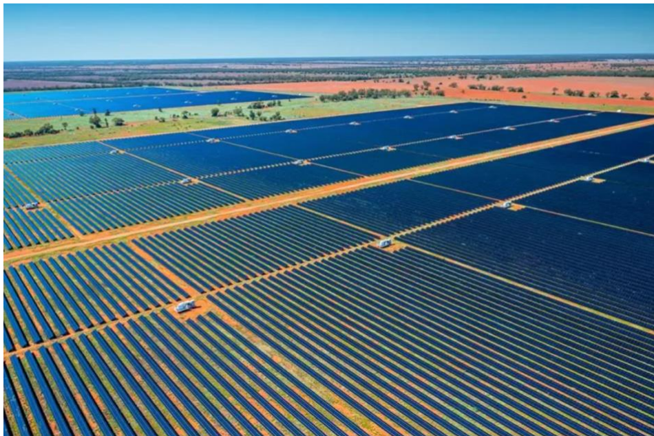
Sudair Solar PV Power Plant
